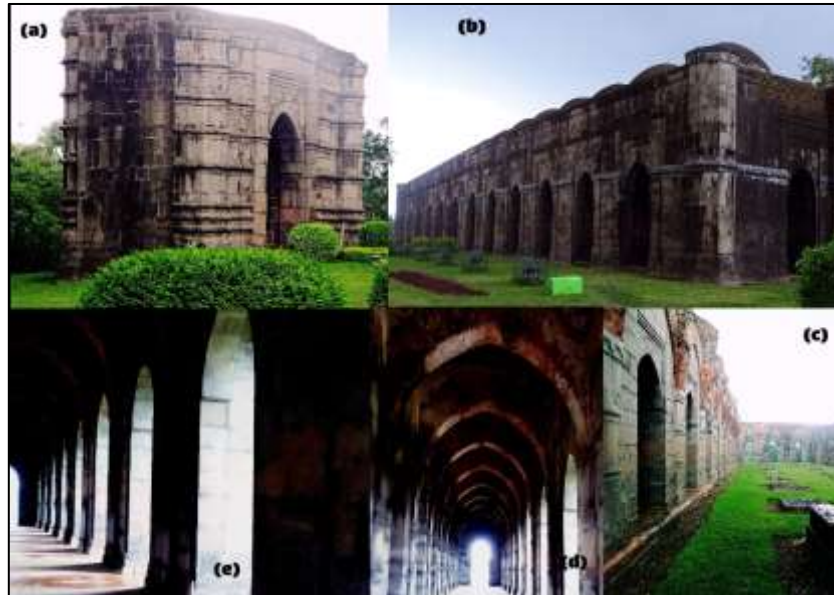
Figure 2. Different portions of Baro Shona Mosque (a) Courtyard gateway, (b) Exterior part, (c) External (interior) wall of the ruined musalla with marks of fallen domes, (d) Arched pattern of the interior portion, (e) Aisle.
