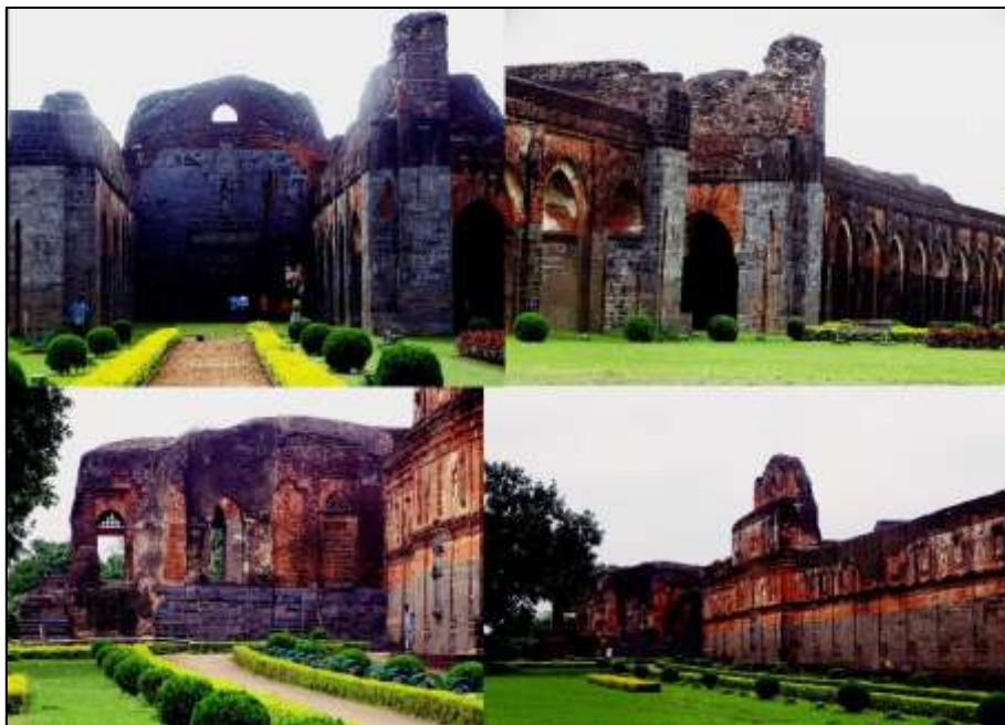
Figure 11. Exterior view of Adina Mosque
