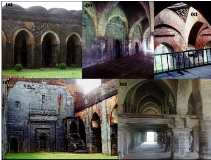
Figure 12. Different Architectural parts of Adina Mosque. (a) Small domes raised over each bay supported by pendentives. These pendentives were formed of brick built in oversailing courses, (b) Mihrabs, (c) Range of arches carried by pillars, (d) Central nave of the sanctuary is in the form of a well-proportioned hall aligned east and west earlier had a barrel vault, (e) Pillars of prayer hall which are Graceful fluted shafts and carried different arches.
